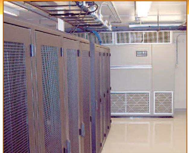
*Server Vault with Liebert air conditioning system, "Unimount" track ceiling, and wire rails eliminate the need for raised flooring expenditures.*
