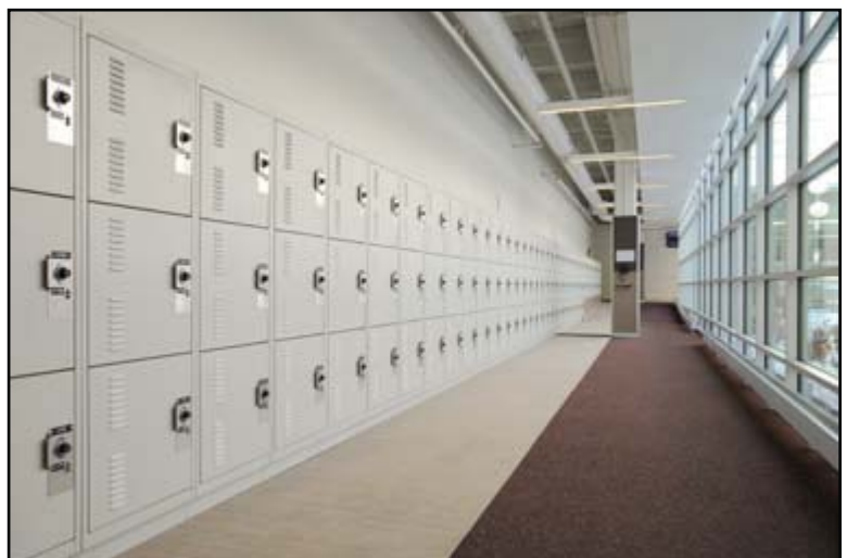
Forty-seven lockers with combination locks designed specifically to store gear bags were installed for the officers use after each shift.
