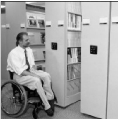
Figure 10. Control guidelines for elevators can be applied to mobile storage. The controls must fall within a height range of 35-48 inches (889 mm-1220 mm) from the floor.
